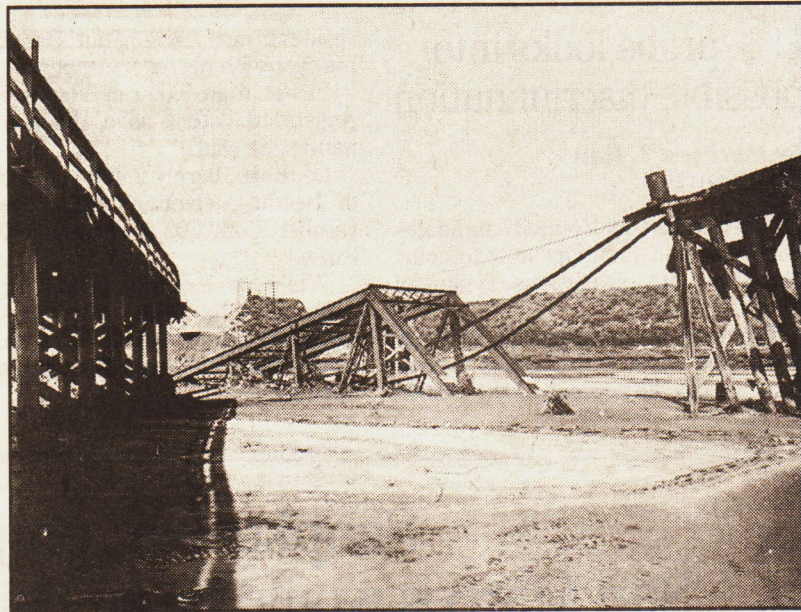
This collapsed bridge contributed to Oceanside being cut off from the rest of the county during the flood. Oceanside Historical Society photos
